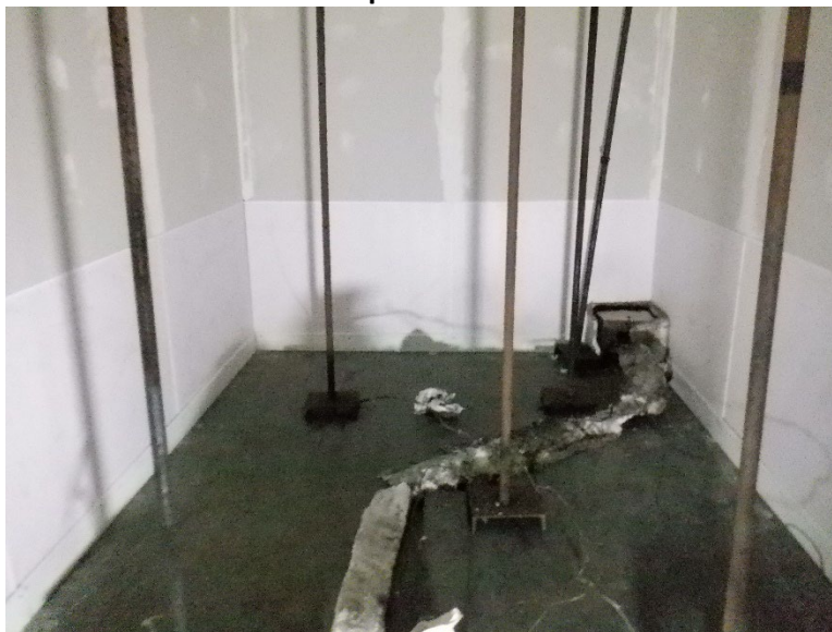
Photo No. 2 Complete Room Pre-test
