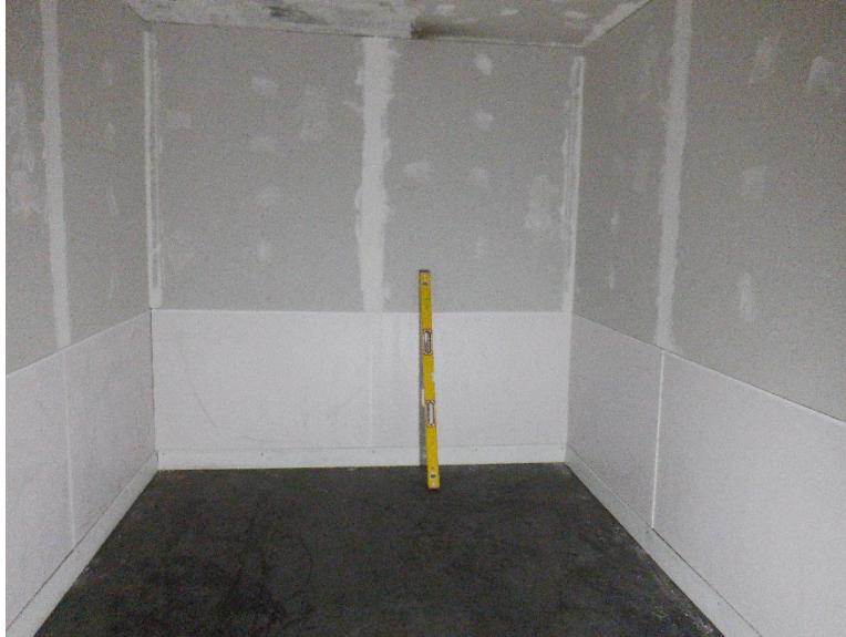
Photo No. 1 Completed Room
